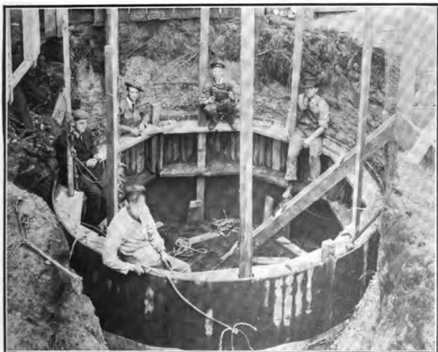
FIG. 2.—STUDENTS OF THE DUNN COUNTY SCHOOL RAISING THE FORM FOR A CONCRETE SILO.
