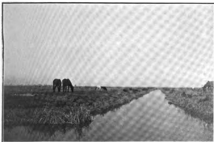
FIG. 2.—EXAMPLE OF A LATERAL DRAINAGE DITCH.
