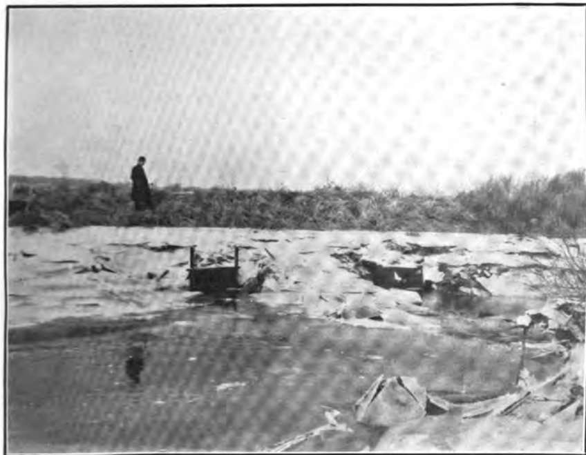
FIG. 1.—SLUICES 8 AND 9, SHOWING FORMATION OF ICE BELOW ORDINARY HIGH WATER MARK.
