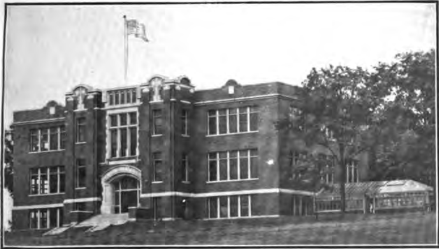
FIG. 1.--MAIN BUILDING, LA CROSSE COUNTY SCHOOL, ONALASKA.
