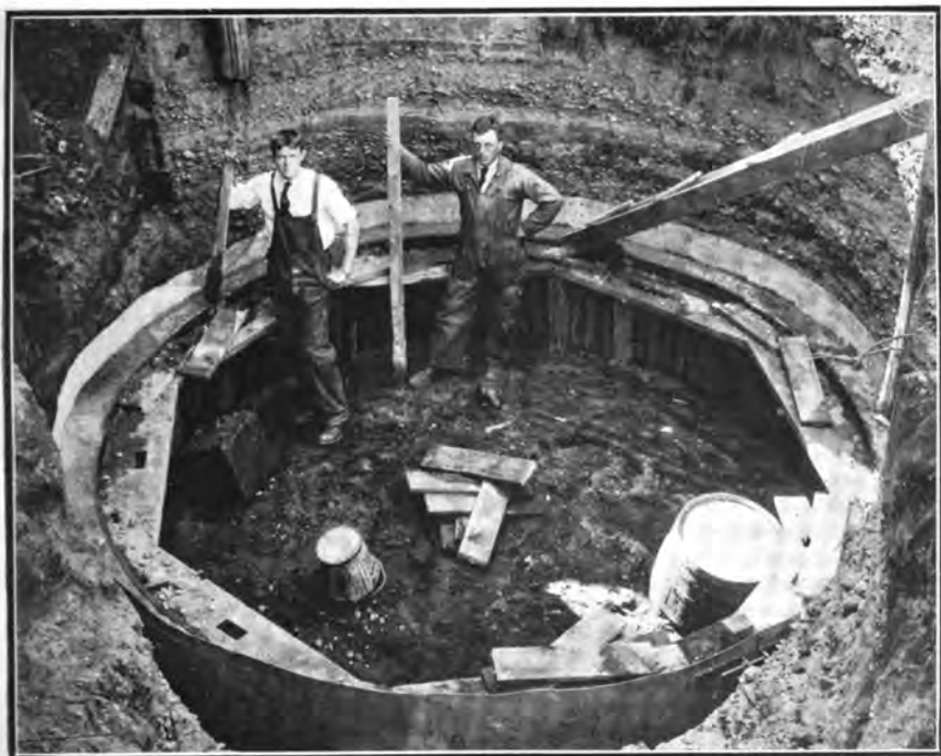
FIG. 1.—STUDENTS OF THE DUNN COUNTY SCHOOL CONSTRUCTING A CONCRETE SILO.
