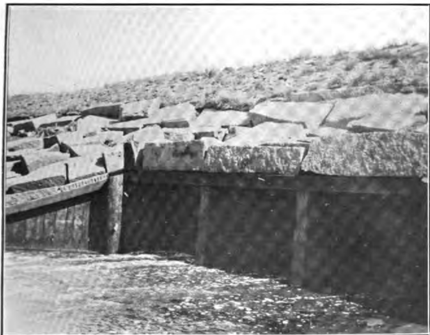
FIG. 1.—OUTER END OF SLUICE AT LOW TIDE, SHOWING GRANITE QUARRY GROUT FACING.
