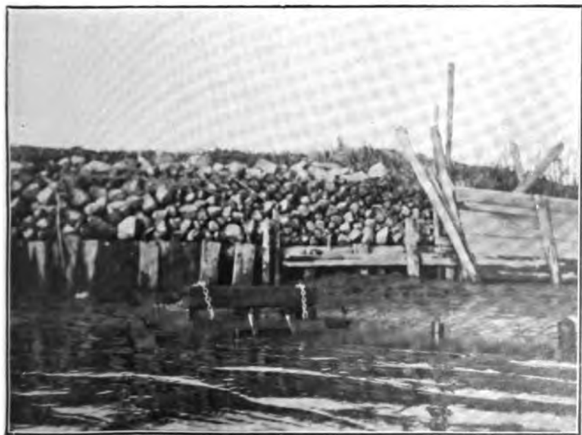
FIG. 2.—METHODS OF LEVEE PROTECTION AND SLUICE 4 AT LOW TIDE IN MAURICE RIVER, DORCHESTER, N. J., NOVEMBER 12, 1909.
