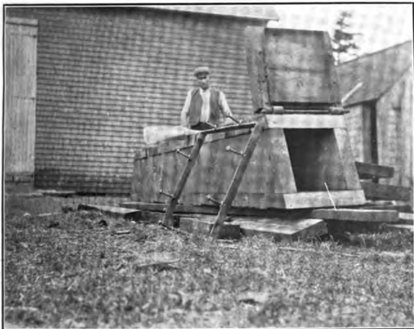
FIG. 1.—SLUICE UNDER CONSTRUCTION AND DEVICE BY ARTHUR A. HICKS, UPPER SACKVILLE, NEW BRUNSWICK, FOR SEALING THE SEAT AND PREVENTING LEAKAGE. [Iron for a larger gate leans against sluice, and a diking spade rests on top.]
