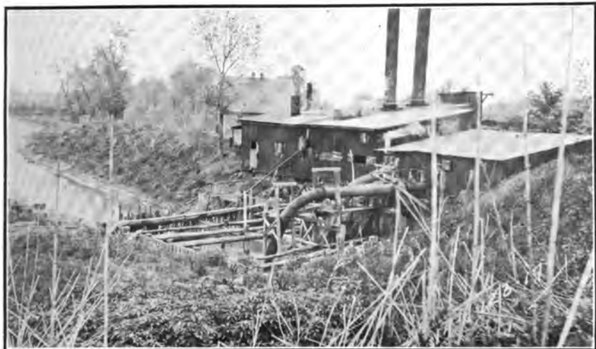
FIG. 1.—PUMPING PLANT, COAL CREEK DRAINAGE AND LEVEE DISTRICT.
