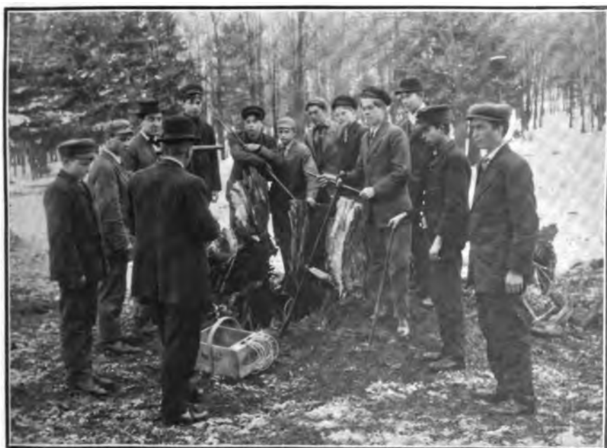
FIG. 2.—MARATHON COUNTY STUDENTS REMOVING STUMPS WITH DYNAMITE.
